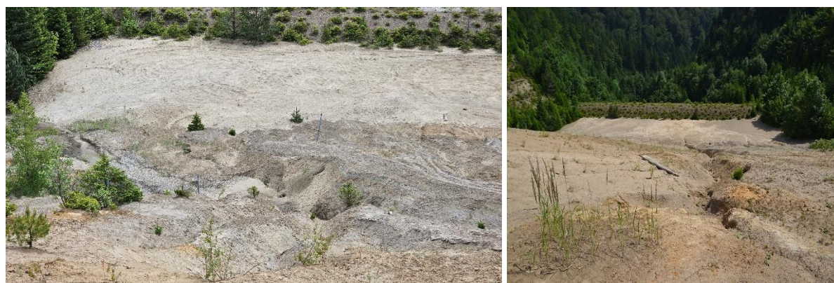
Figure 7. Erosion on the flotation tailings dam
