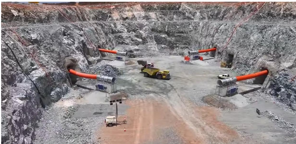
Figure 9. Combination of underground and surface mining with the opening of underground rooms from the pit crater floor level at open pit mine in Kathleen Valley, Australia
