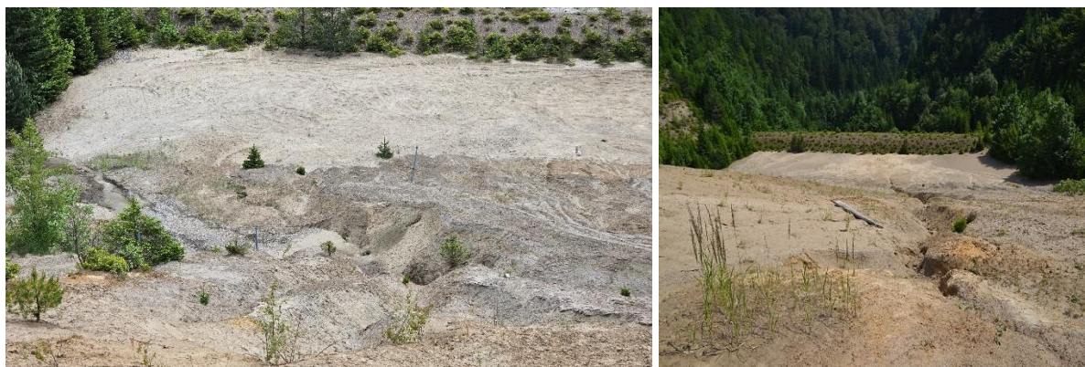
Figure 7. Erosion on the flotation tailings dam
