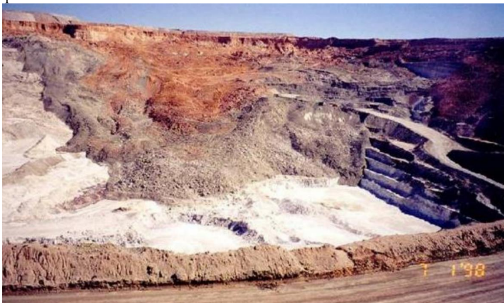
Figure 1. Landslide at the Rio Tinto open pit mine in the Mojave Desert in the Kern region near Los Angeles in 1998
