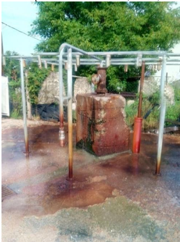
Figure 3. View of the mouth of the borehole SI-1 in Slavinovici, with the construction of the choke manifold (showers) (Photo: Nuhanovic, S; Barusic, B., 2020.)
