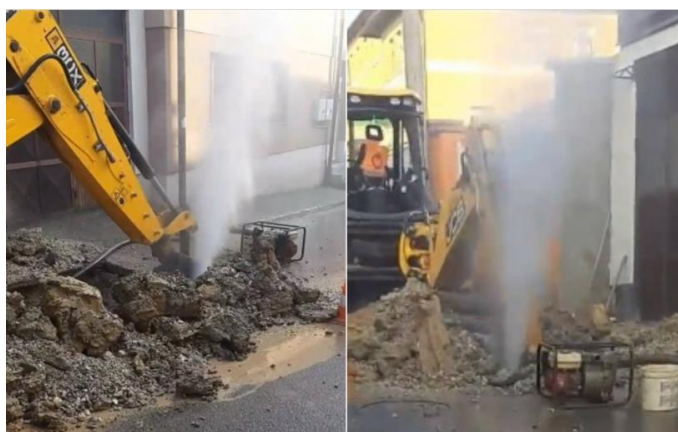
Figure 5. Damaged gas pipe (Source: https://www.faktor.ba )
