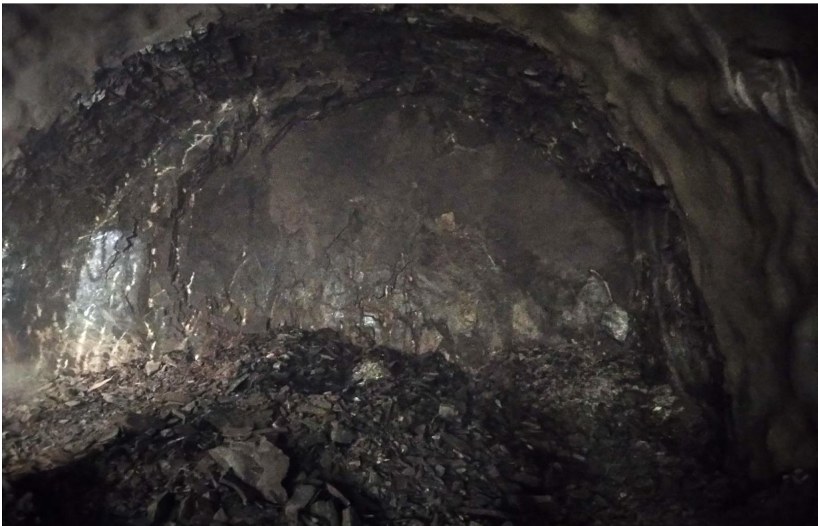
Figure 10. LTT face cross section at chainage 1+524.088 after blasting and treatment of the cross section
