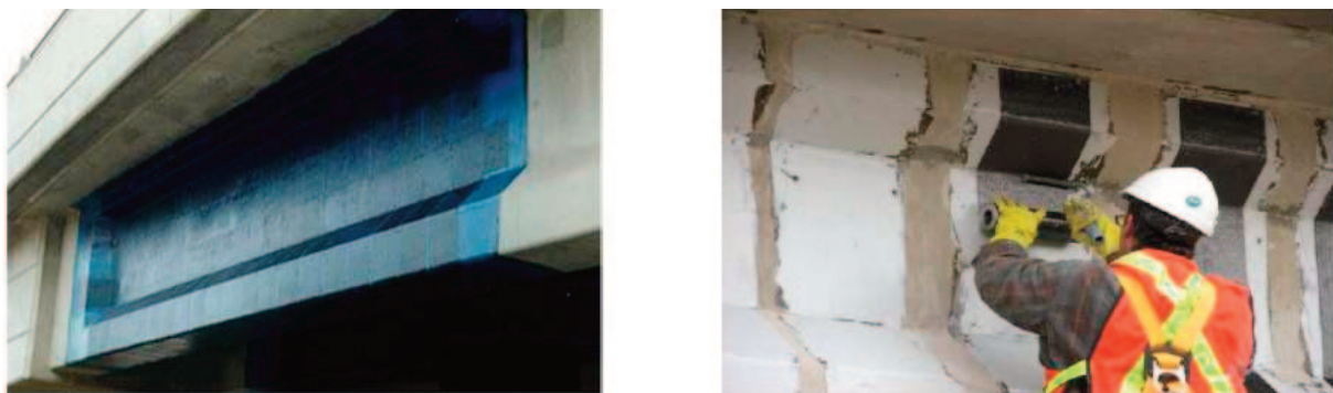
Figure 1. Strengthening of the RC structure using carbon (CFRP) strips [4]
